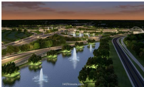
I-4 Ultimate Project, Central Florida
