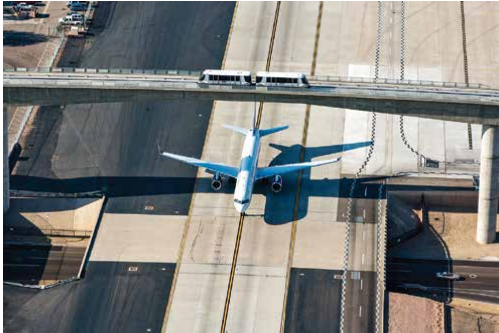
The development of the PHX Sky Train required several unique design features, including the world's first transit bridge over an active taxiway.
